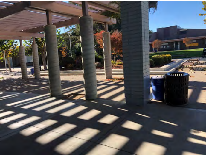
Western Side of Gymnasium – Facing West
