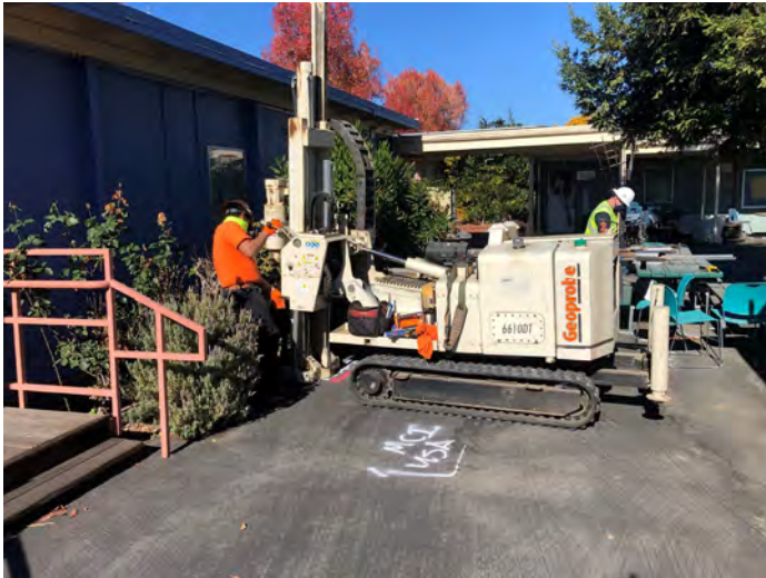
Drilling NOA -8 Central Portion of the Freestyle Academy
