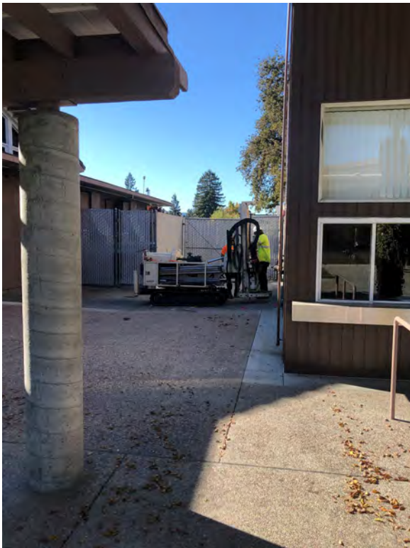
Sampling Southern Side of Cafeteria
