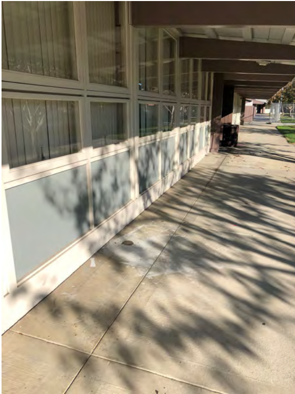
Coring Southern Side of 100 Block
