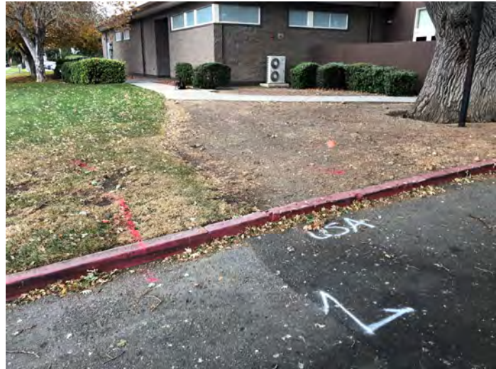
Western Side of Cafeteria – Facing Northwest
