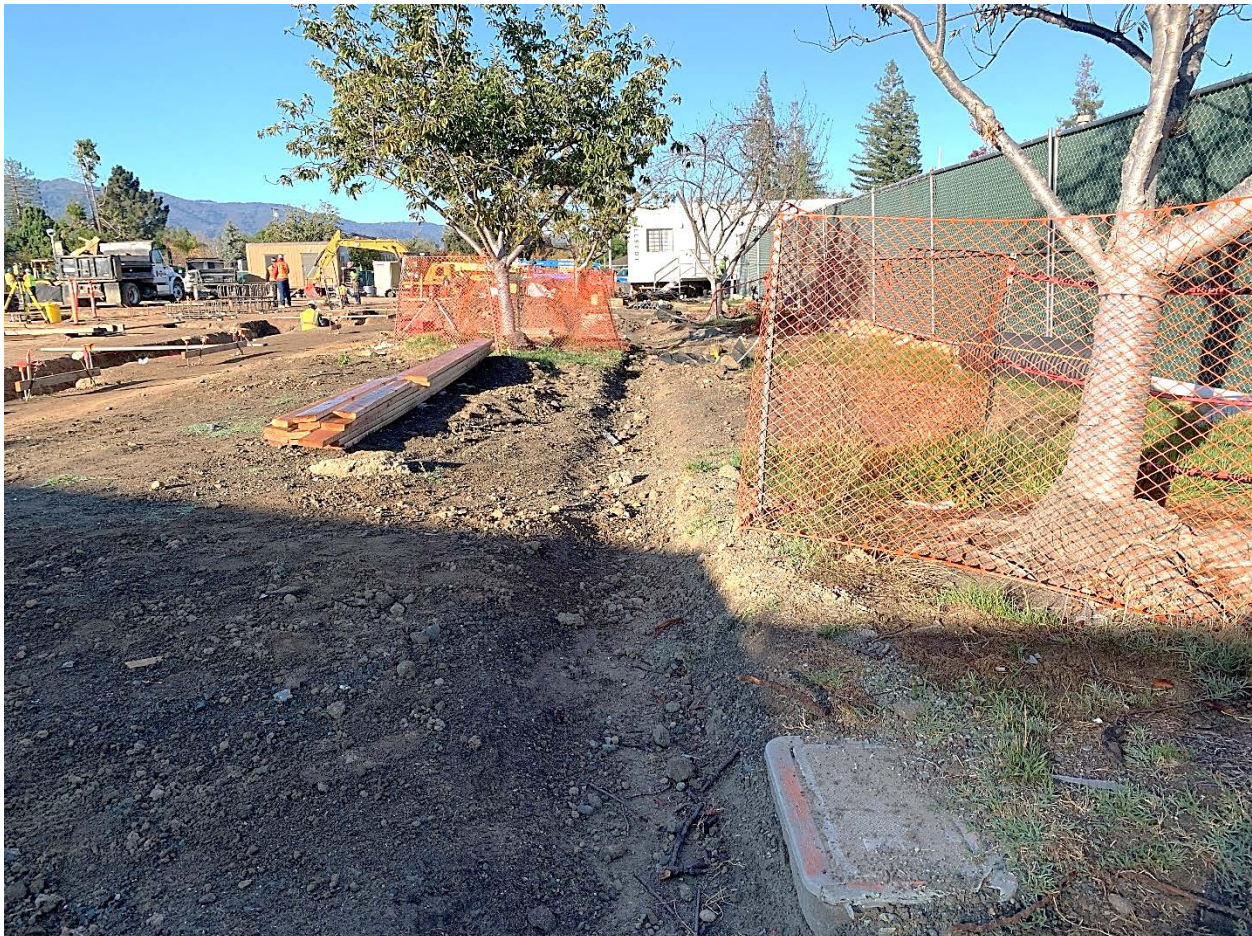
Image #10, - Trees T1, T2, T3 & T4, cherry. Note linear soil depression from pipeline installation.
