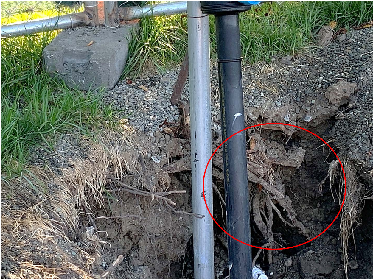
Image #9, - Tree T5, cherry. Several one half to 1" diameter roots were cut for tie-in, (circled).
