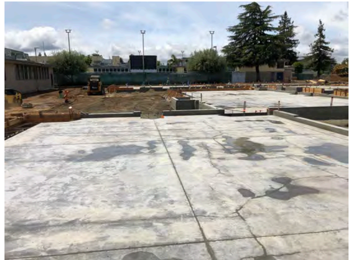
New Foundation in the area of former 600 Building
