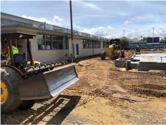
Grading North of the 500 Building
